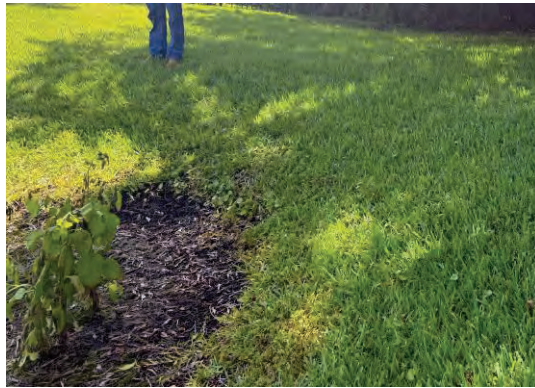
North side lake slope appears to be greater than 4 to 1 This area is not safe
