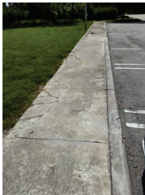
Damaged Curb and sidewalk on the north side of the parking lot just east of Laceleaf Court
