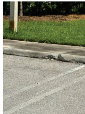
Damaged Curb and sidewalk on the north side of the parking lot just east of Laceleaf Court
