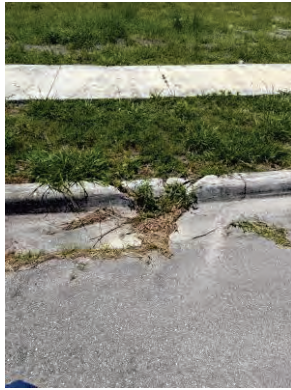
Damaged curb and unfinished sidewalk on Baneberry Lane in between lots 19 and 20
