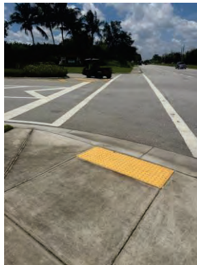
Striping present within Right-of-Way; Onsite striping not present or is overall faded
