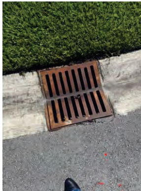
New Catch Basin on Eagle Oaks Lane. This will be identified as 92 on reports from here on.
