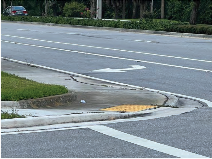
ADA curb ramp on Congress Ave
