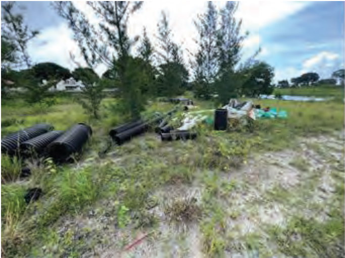
West Embankment of L-1 – Material storage area
