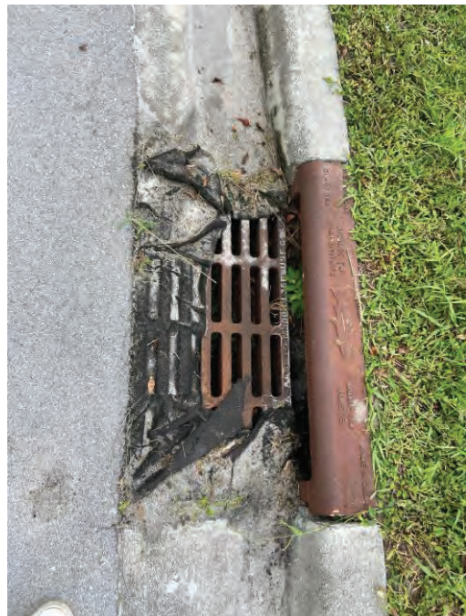
Catch Basin on the side of Banyan Club Rd (typical)
