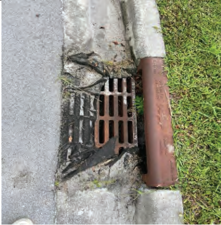
Catch Basin on the side of Banyan Club Rd
