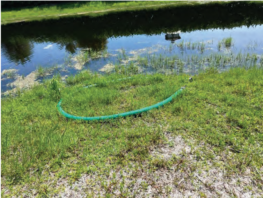
Tube on SE end of L-3 Embankment
