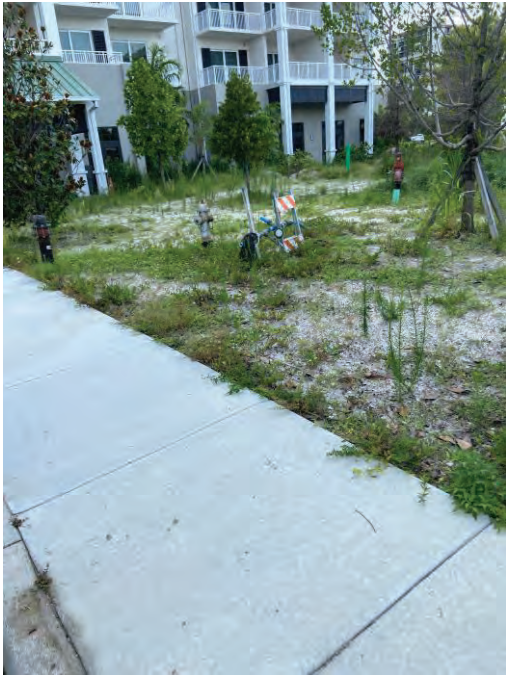
Unstable backflow preventer NE of the garage entrance
