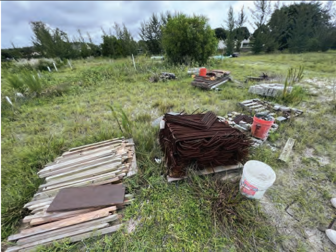
Unused material stored East of the Banyan Villa Circle
