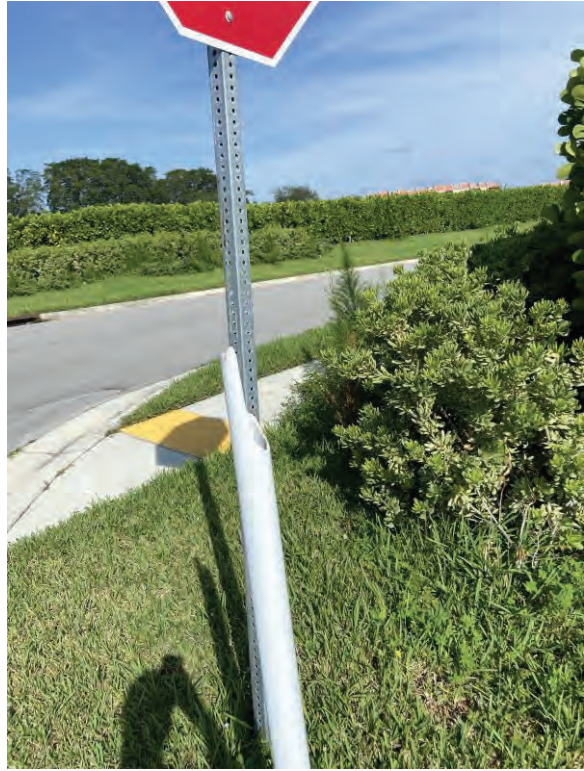
Sharp edged standing pipe on a side of Terranova Ave
