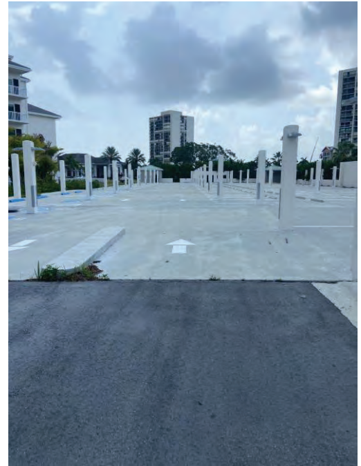
Parking Garage Entrance
