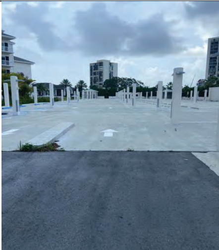
Parking Garage Entrance
