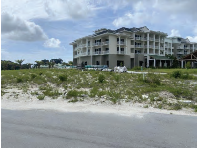
Banyan Villa Circle – Dirt leaking on the road due to lack of maintenance
